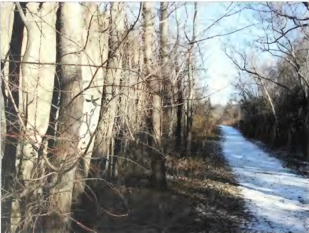
Figure 5.74. View looking northwest along interior trail, the Mortar Battery. Given the harmful effect of woody vegetation growing in close proximity to concrete structures, all woody vegetation growing on or within four feet of concrete features should be removed (Olmsted Center, January 2009).
